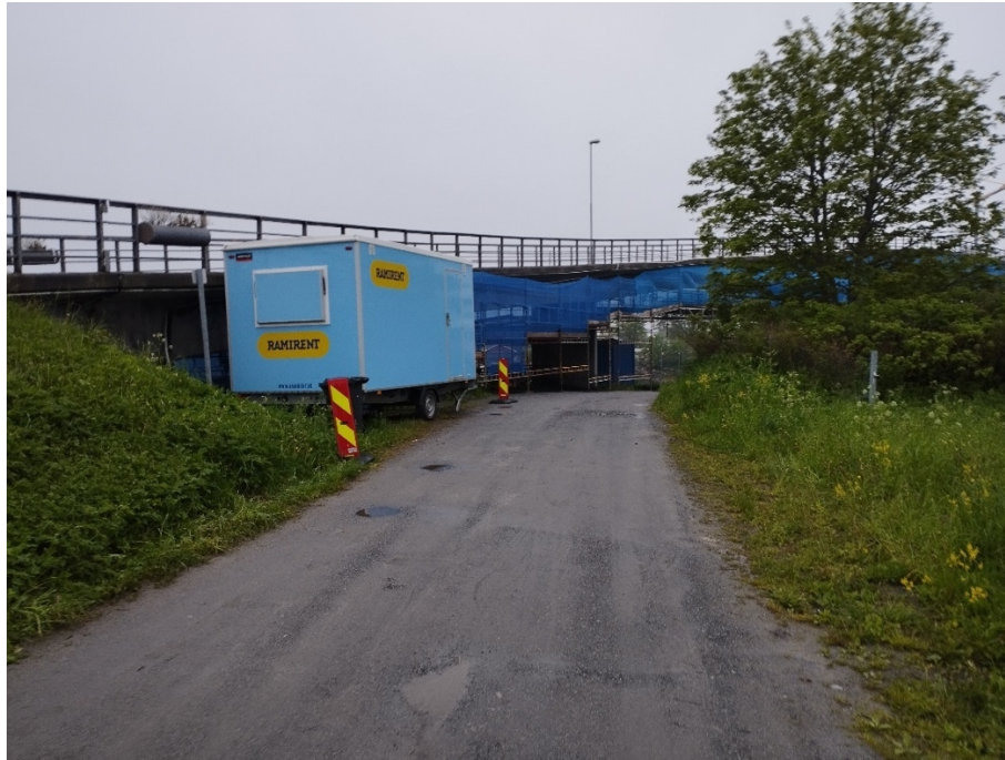
Fig. 44 Cabin office by the bridge.
