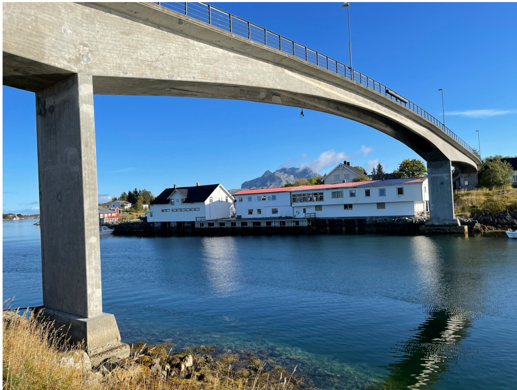
Fig. 7 Picture of Herøysund bridge.
