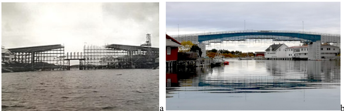
Fig. 50 a) Construction phase (1966), b) upgrading work (2020) ( https://www.wikiwand.com/no/Herøysundet_bru ).
